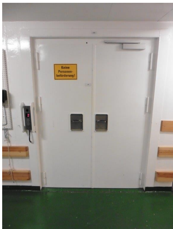
Goods lift (main deck level) closed
